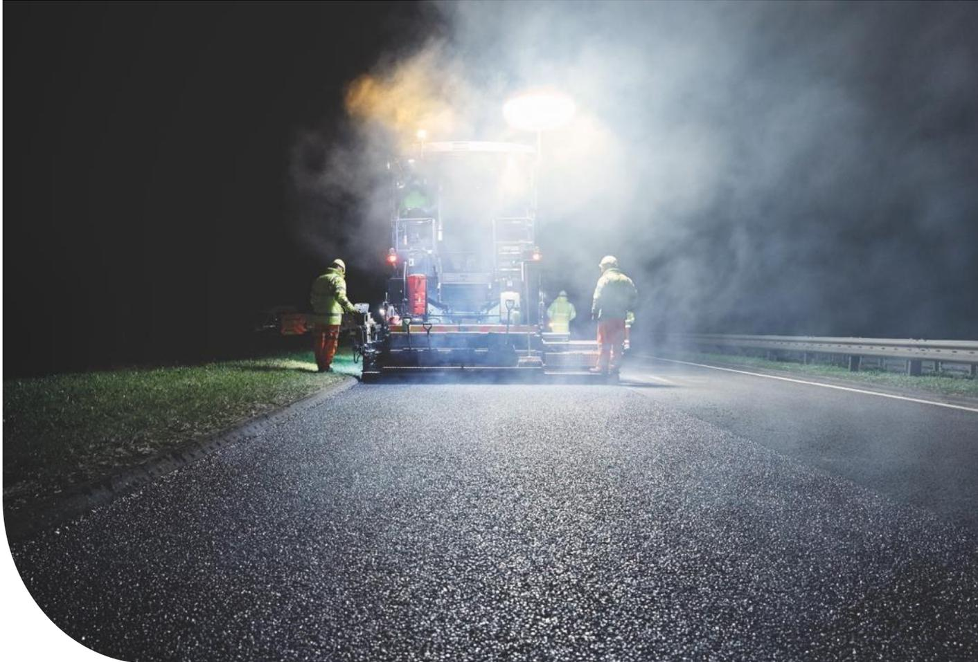
We are trialling asphalt containing additives derived from waste plastics in a project with Cumbria County Council aimed at reducing the carbon footprint of highways schemes and providing a more resilient road network.
