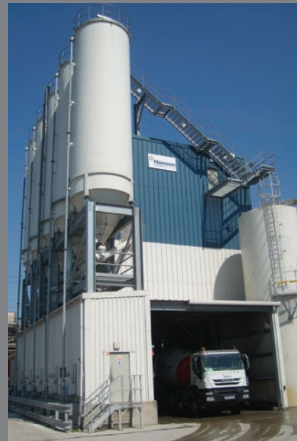
Silvertown concrete plant in London.
