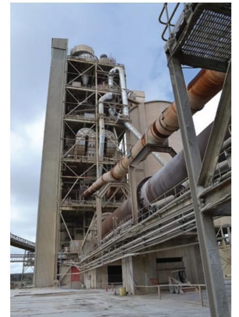
The main kiln at Ketton cement works in Rutland.
