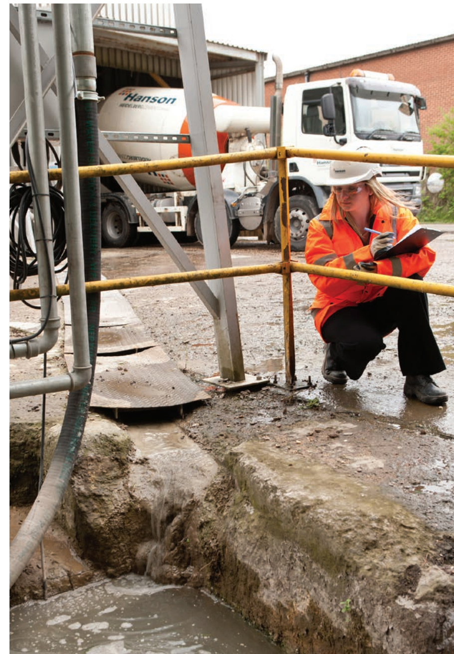
IMS coordinator Gemma Leavesley inspects the process and storm water recycling system at Tile Hill ready-mixed concrete plant in Coventry.
