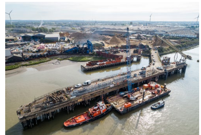
Dagenham aggregates depot
