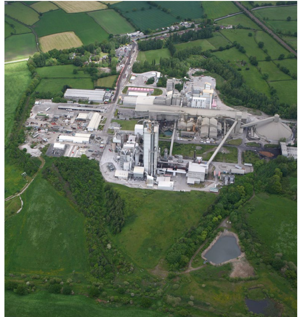
Padeswood cement plant in Mold, Flintshire
