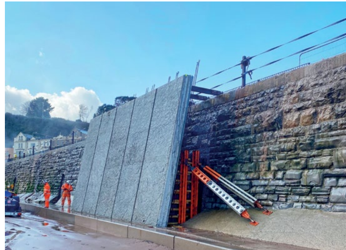
Coastal protection works in Dawlish, Devon
